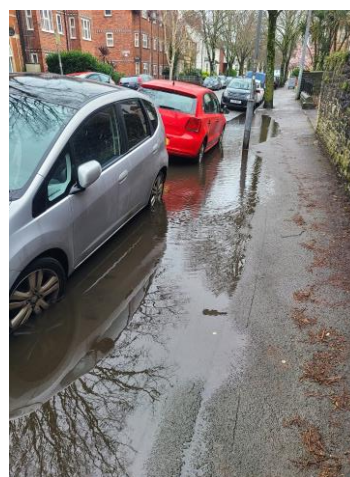
Localised gullies/drains blocking
