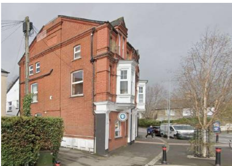
The Old Bakery frontage
